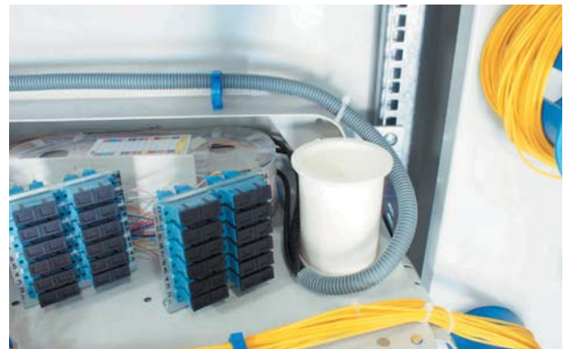
Splicing will be done inside high density cassettes
