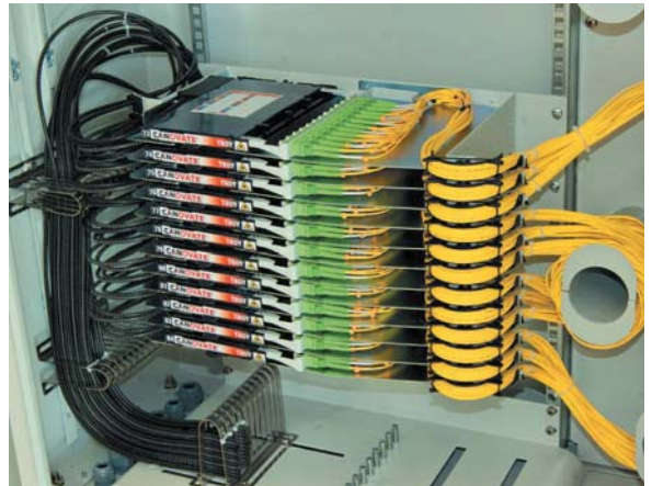
Each U accommodates 2 fiber trays Integrated patchcord mandrels 19" rear mountable
