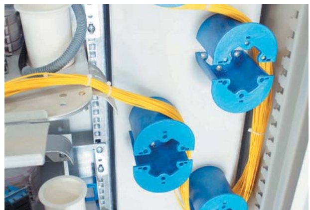
Excess cables are stored via special bendradien to ensure required bending criterias
