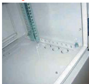
Fiber cable hole entries for telecom cables from underground
