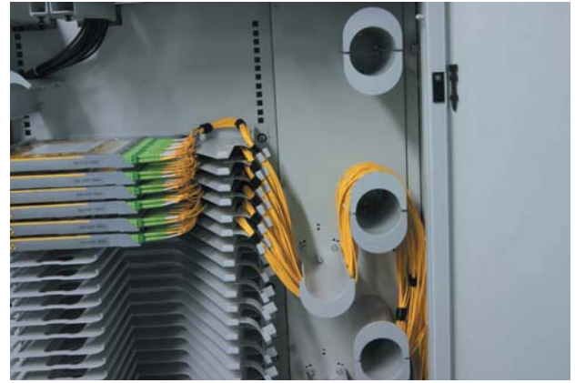
Patchcord Routing Guides
