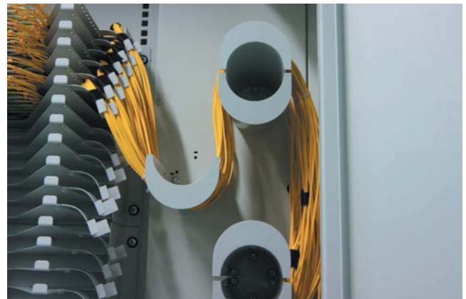
Patchcord Storage Area
