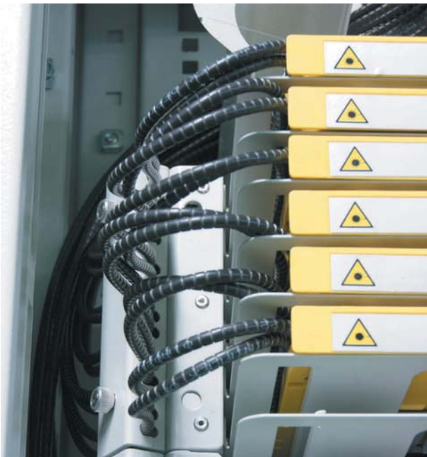
Miniflex tube entry inside the ODF modules
