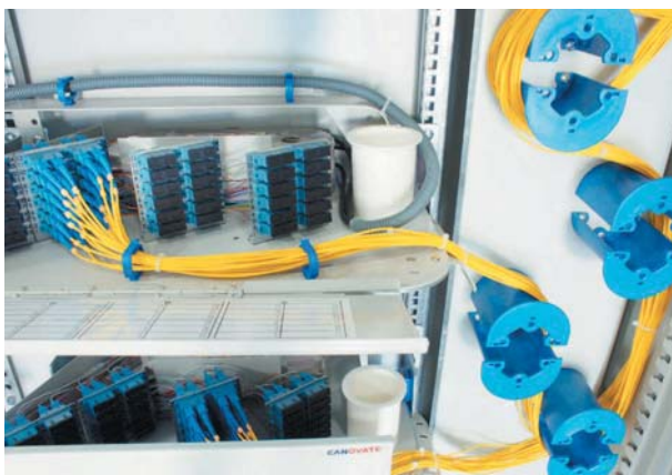
Patchcords are routed via cable holders to the excess cable storage area
