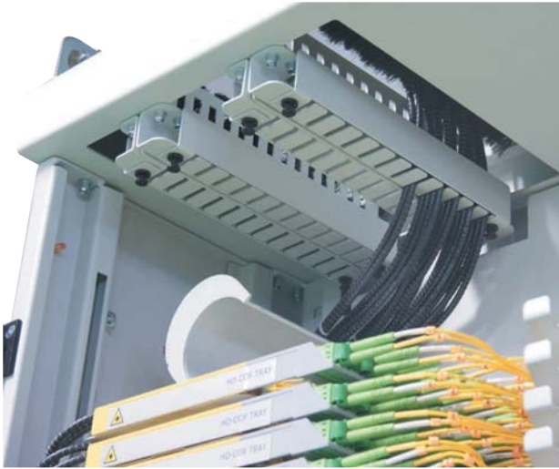
Incoming Cable management with miniflex tubes
